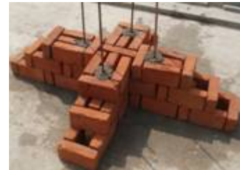
Reinforced Cross- Junction
