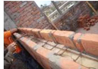
Reinforced Sill or Lintel Band
