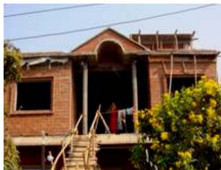
Residence at Butwal
