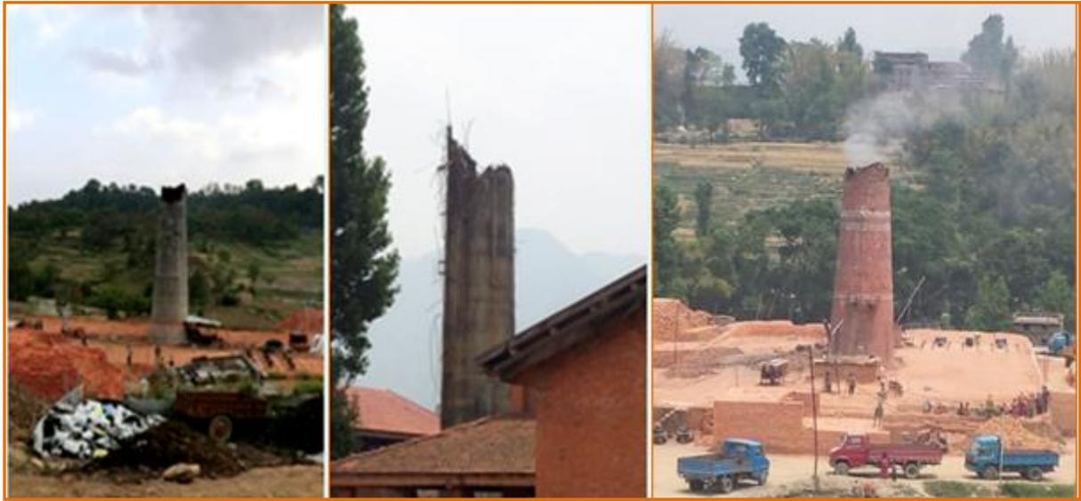
From L to R: FCBTK kiln in Lalitpur, Hoffman kiln in Bhaktapur, and FCBTK in Bhaktapur. All were damaged by the April 25<sup>th</sup> 2015 earthquake.
